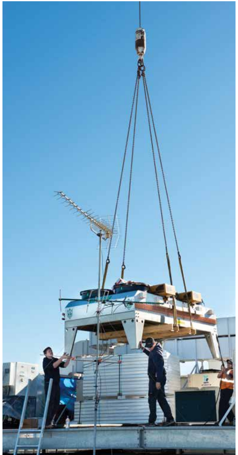
The new refrigeration system being installed on the roof of the Lidcombe Club
