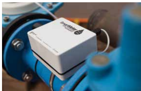
The new smart metering system at Lidcombe provides energy usage data in real time
