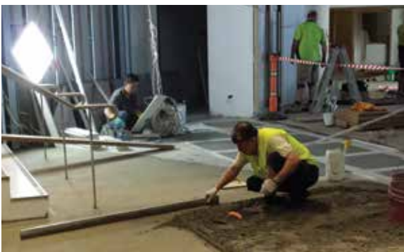
Renovations to the Church Street foyer concluded in June 2014
