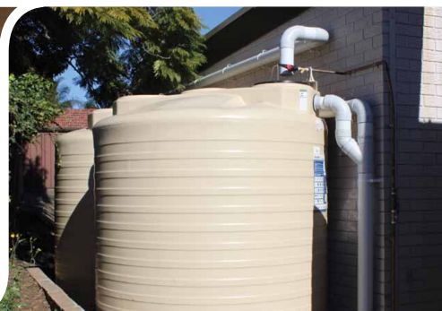
Rainwater Tanks
